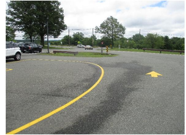
Pervious pavement can be installed in the southernmost row of the parking lot to capture, treat, and infiltrate stormwater runoff from the parking lot. A preliminary soil assessment suggests that the soils have suitable drainage characteristics for green infrastructure
