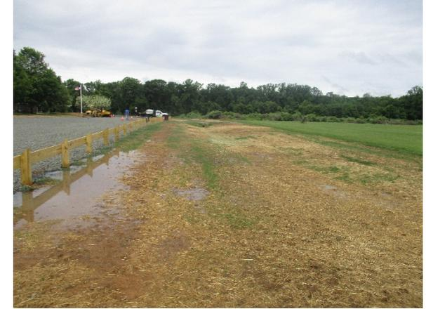
A rain garden can be installed along the northern edge of the parking lot area to help infiltrate the pooling stormwater in that area. A preliminary soil assessment suggests that the soils have suitable drainage characteristics for green infrastructure.
